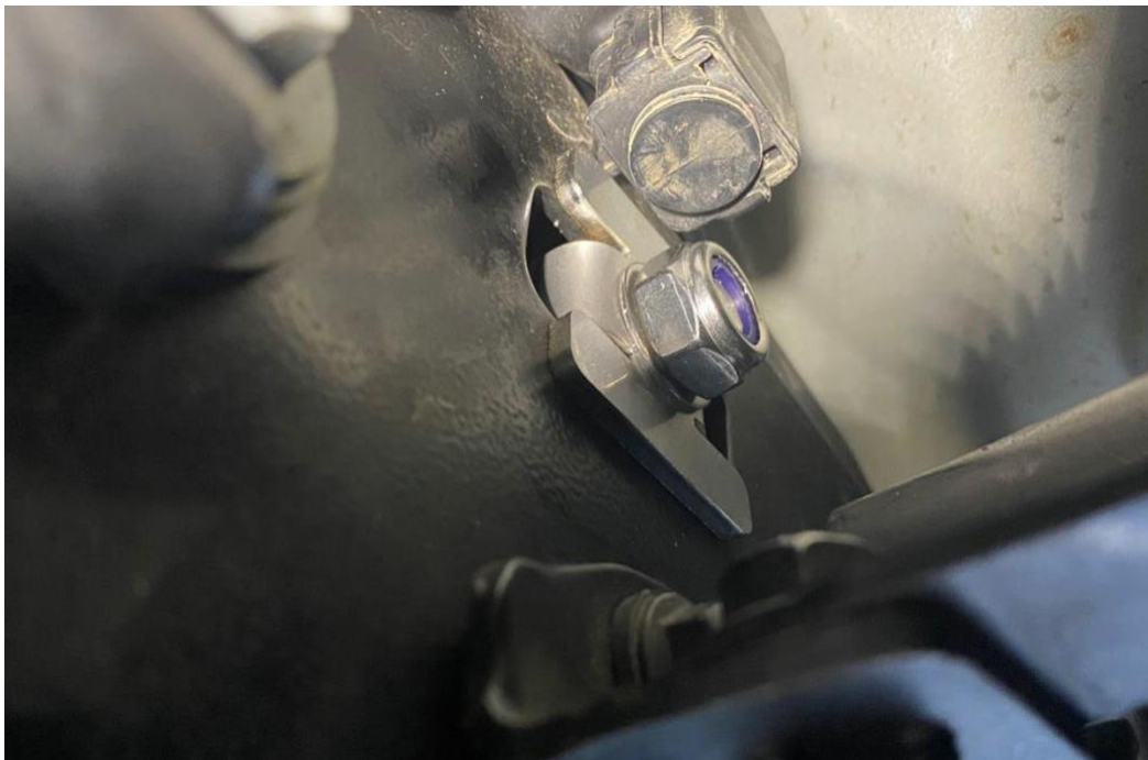
Inside view of new bracket secured in place
